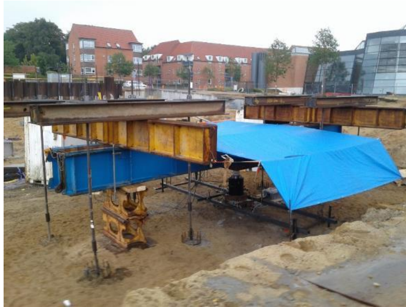
Figure 4. The test setup.
